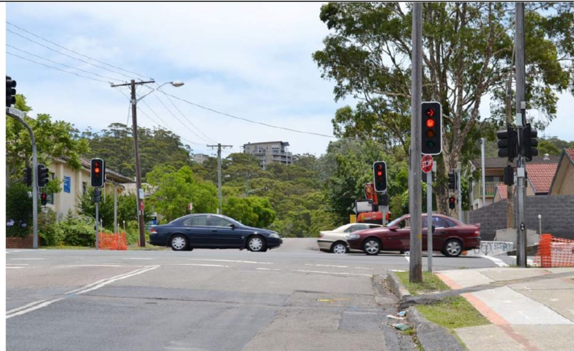
Figure 5.3.3 View from the intersection of Frederick Street and the Central Coast Highway
